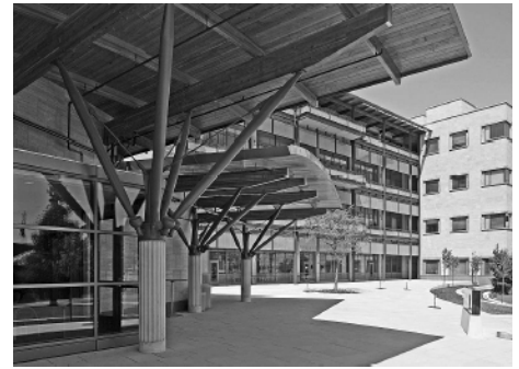
UCSD Biomedical Research Bldg: Tree columns supporting entry canopies.
