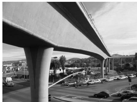
Mission Valley Bridge: At Mission Gorge Road.
