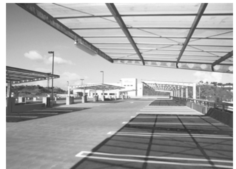
Kaiser Parking Structure: Rooftop parking.
